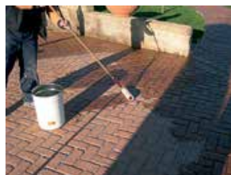
8. Aplicarea rasinii Sealfloor 100
