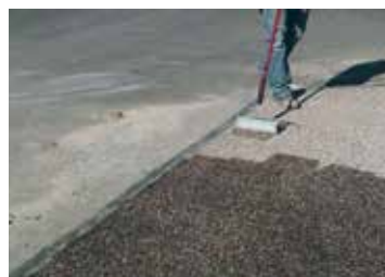
5. Aplicarea rasinii Sealfloor 100
